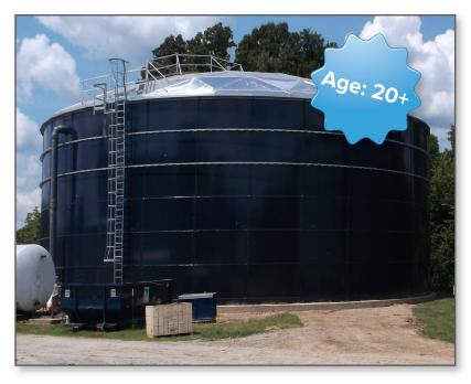
Dave Hemauer, project manager at Cady Aquastore. "But it took only nine days after the tank was drained and washed out to rehab and make improvements to the older Aquastore tank. After a few days of sealer curing time, the tank was ready for sanitizing and bacteriological testing and back in service."
