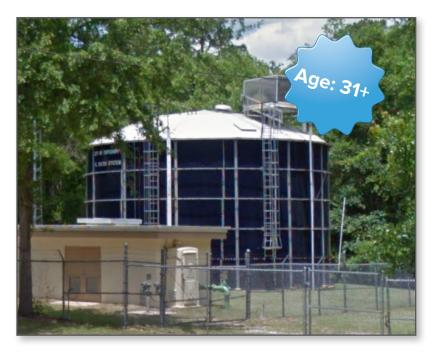
durability, appearance and the low cost of maintenance. "The Aquastore tank has more than performed as advertised in every aspect," says Tartt. "By comparison, the steel tanks fade over time and need to be repainted and they need more repair than the Aquastore."
