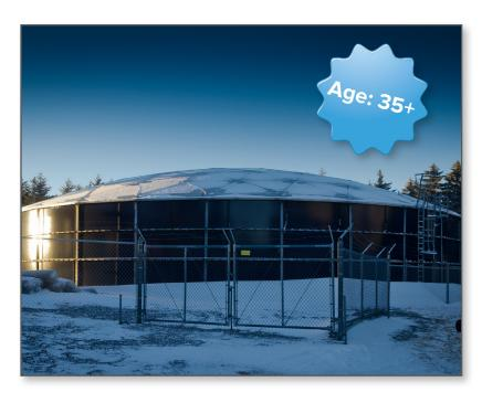
In 2009 when the water company moved overflows and installed replacement sheets, it was surprised to find upon inspection that the interior of the 35-year old Aquastore tank was in near perfect condition.
