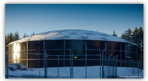
The challenging climate also makes it surprising to find that the Water Plant's oldest potable water tank, an Aquastore tank provided by Mid Atlantic Storage Systems capable of storage for 500,000 gallons recently celebrated 35 years in service without significant maintenance.
