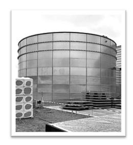
When the above challenge was coupled with a very tight deadline to manufacture, supply, and install; it led to only one solution - A single tank. Except at this size there were few options available. Fortunately, CST has pre-approved FM tank sizes ranging from 57m3 to 2,548m (15,057 to 673,110 US Gallons) and was able to manufacture and install the tank within 10 weeks.
