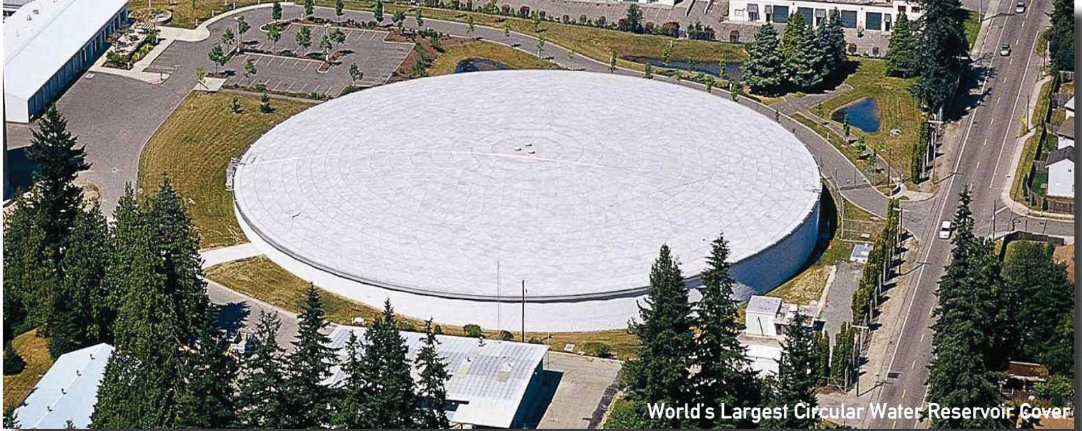
Alderwood Water & Wastewater District Lynnwood, Washington - 375' diameter
