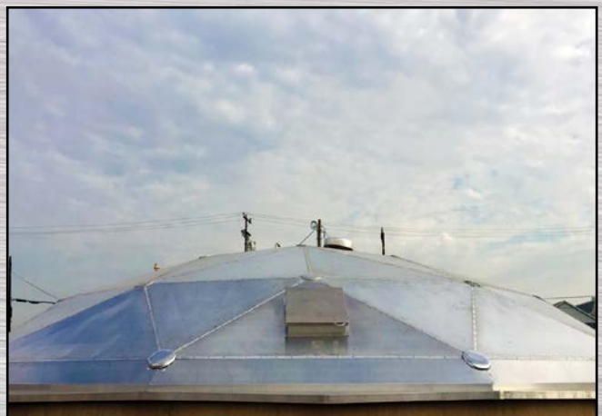
Golden State Water Company Huntington, California - 60' diameter
