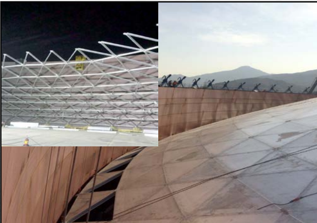
National Water Company Makkah, Saudi Arabia - 361' diameter
