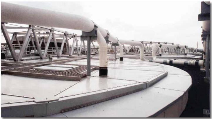
(8) 75' dia. truss supported flat covers Sayreville, NJ 1994 Engineer: Montgomery Watson Engineers
